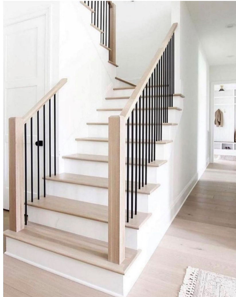
STAINED SQUARE NEWEL POST AND HANDRAIL WITH IRON SPINDLES
