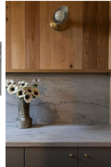
COUNTERTOP BACKSPLASH UP TO BOTTOM OF UPPER CABINETS (SEE RED LINE) WITH COUNTER LEDGE BEHIND RANGE AND WOOD PANELING ABOVE AND AROUND WINDOWS
